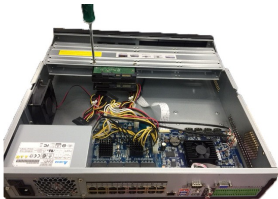
Figure 15-15 Placing the HDD
